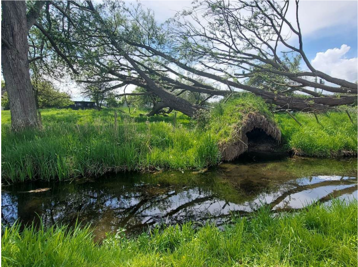
Figure 2-5 Overview of the WC5.
